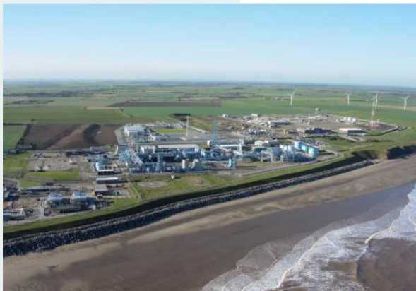
Easington Facility, Centrica
